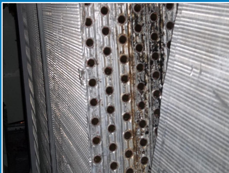
CROSS SECTION OF COIL
